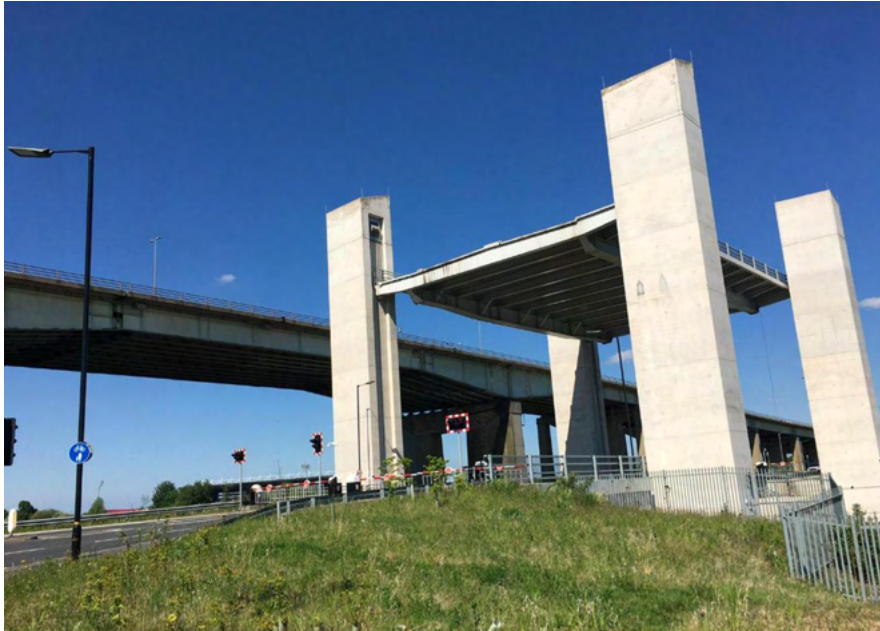
Dom waits for the A57 Barton Lift Bridge to descend while his mum tries to catch him up!
